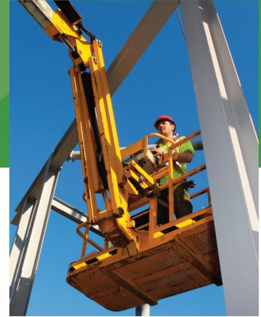
Improper use of access equipment on construction projects continues to cause workplace injuries in Ontario. The use of elevating working platforms may put workers at risk when the equipment is not adequately used, maintained or stored, or when manufacturer's instructions are not followed and equipment limitations are not respected.
